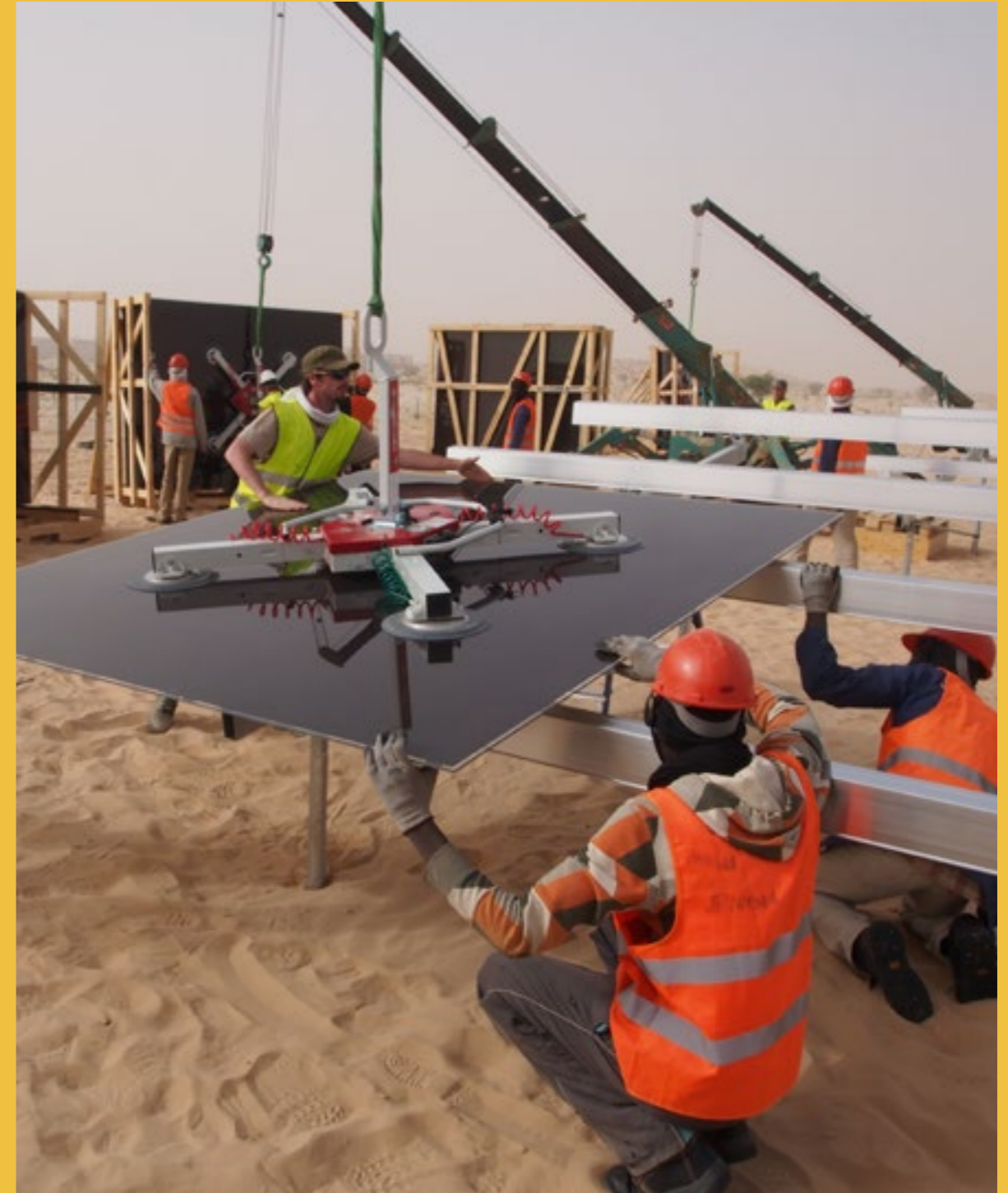
Building the Mauritania solar plant
