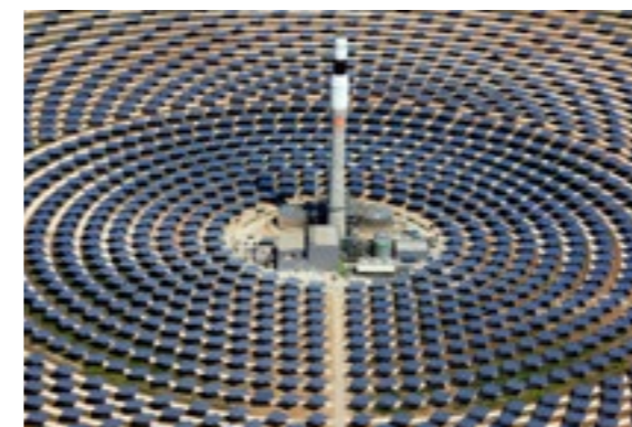
Gemasolar 19.9MW CSP Plant in Seville, Spain
