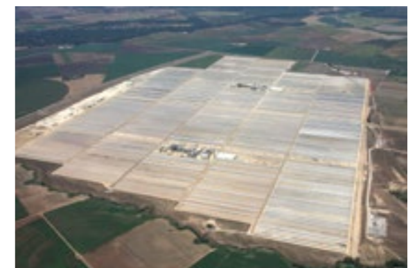
Aerial view of Valle 1 and Valle 2, adjacent solar plants that generate electricity by means of cylindrical-parabolic collectors
